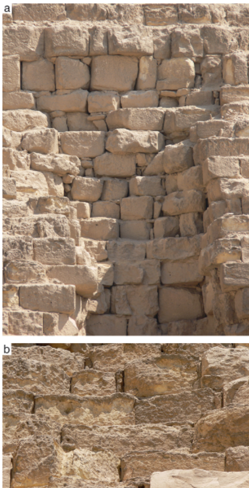
Fig. 6. Photographs of (a) Vyse's gash in Khufu's south face. It is clear that these blocks were most probably not cast, (b) blocks just below the gash; these appear to have been cast.
